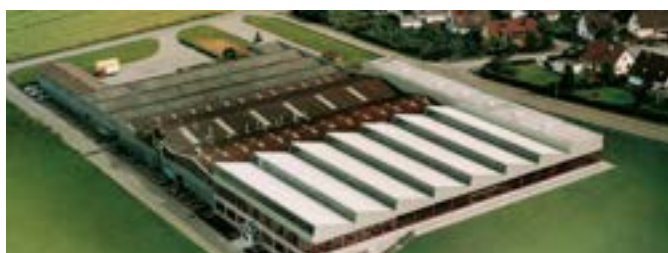
Häfele Production Plant Jettingen, Germany
