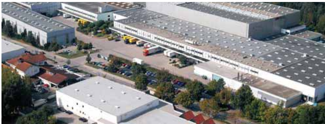
Häfele Distribution Centre Nagold, Germany
