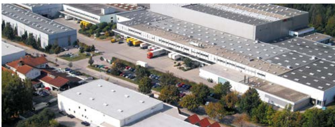
Häfele Distribution Centre Nagold, Germany
