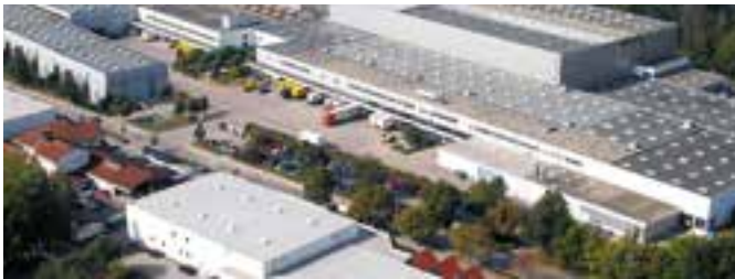
Häfele Distribution Centre Nagold, Germany
