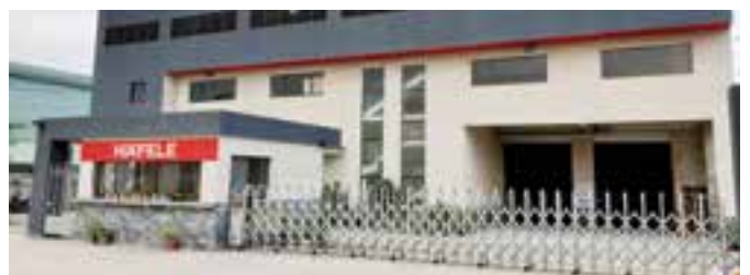
Häfele Production Plant Binh Duong, Vietnam
